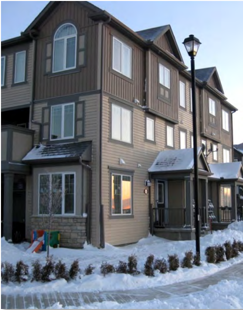
Photo: 2 - Example of Multi-unit development with prominent street frontage in Airdrie, AB. Source: ORRSC
