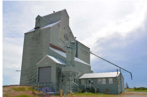
Figure 6 - 2020 photograph of the Alberta Wheat Pool Grain Elevator in Fort Macleod (Promethean Heritage).
