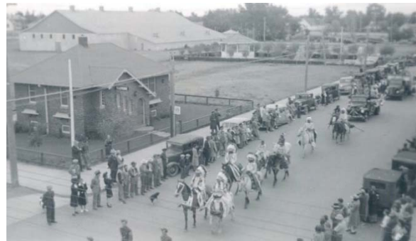
Figure 3 - Telephone Exchange Building seen in this parade photograph (Fort Archives FMP 81.145.5).
